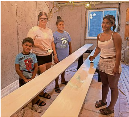
Habitat for Humanity of Fond du Lac County's partner family for this year's home build is Amanda Buechel and her family, pictured here painting the trim for their future house. PROVIDED BY HABITAT FOR HUMANITY OF FOND DU LAC COUNTY
