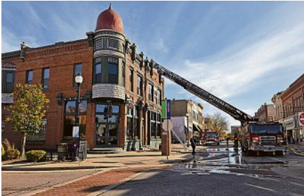
Emergency crews responded Oct. 9 to a report of a structure fire on the second floor at 912 Main Street or Graffiti’s Sports Pub. ERIK PFANTZ/STEVENS POINT JOURNAL
