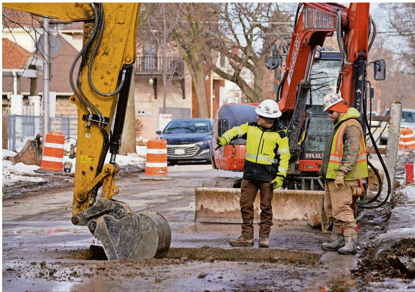
Chris Williams, left, and Eddie Christoffel, Milwaukee Water Works foreman, work in the 2000 block of North 49th Street, where lead pipes are being replaced with copper pipes. PHOTOS BY ANGELA PETERSON/MILWAUKEE JOURNAL SENTINEL
