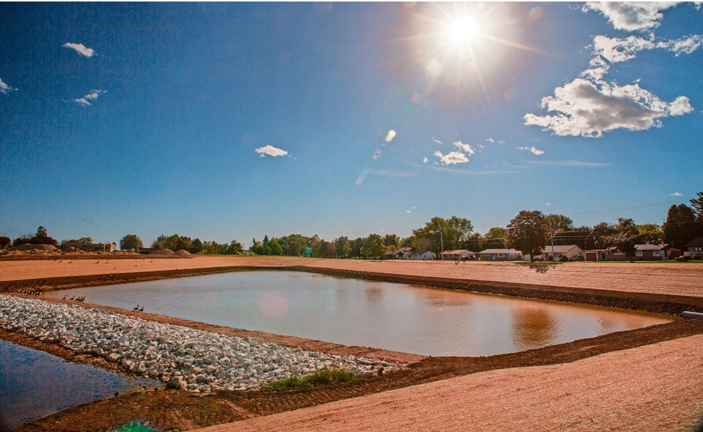
The sun shines above a retention pond that is nearly complete at the Mariner Lux Subdivision as seen Oct. 7. The subdivision is being built where Mid-Cities Mall and Edgewater Plaza once stood.
