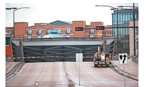
The Main Street bridge will be closed from June 4-25.
