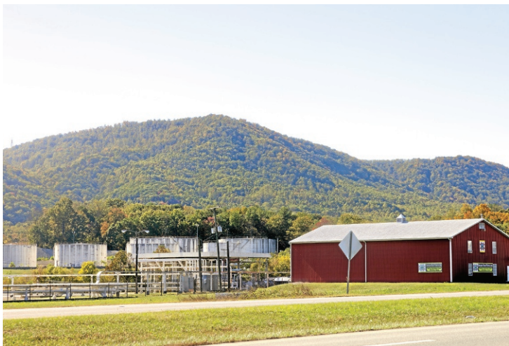
The 140-acre tank farm’s status is closed with 35 tanks and 47.5 million gallons of capacity.
