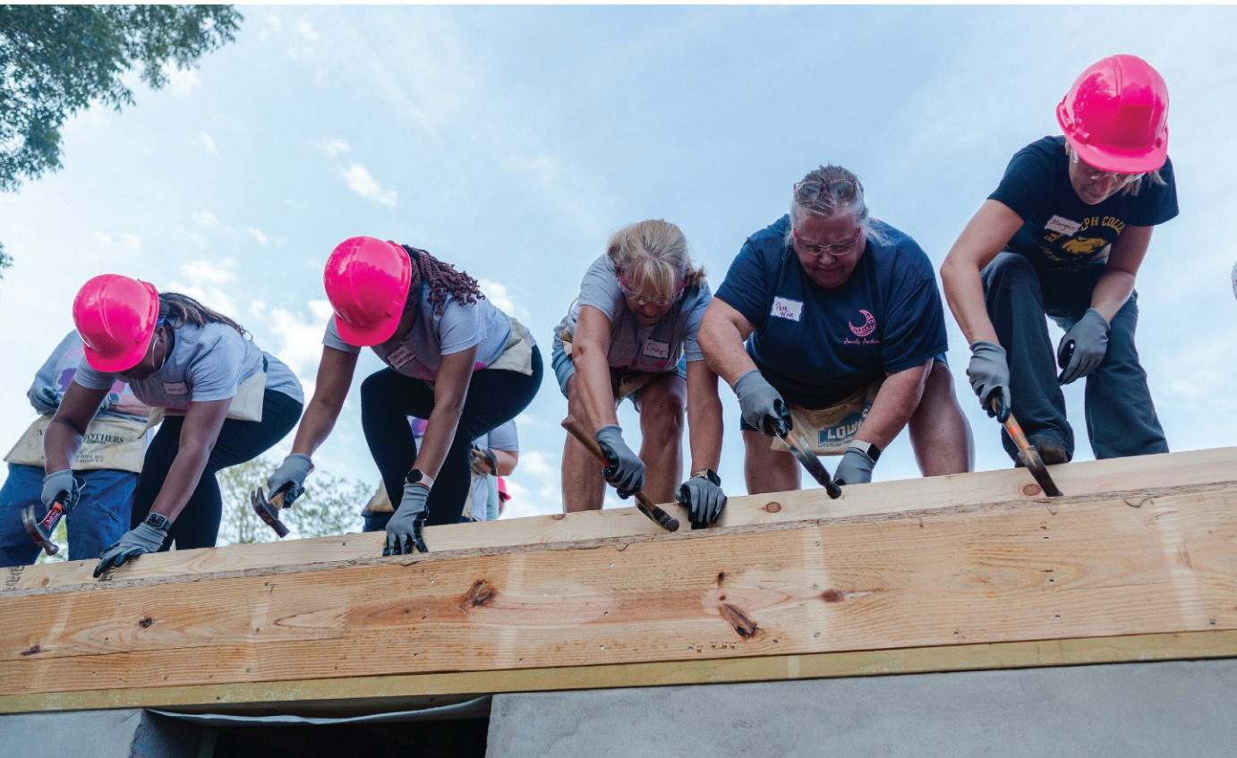
MATTHEW PERSCHALL PHOTOS, THE NEWS & ADVANCE Volunteers help construct a wall as part of Lynchburg Habitat for Humanity's Women Build initiative Saturday.
