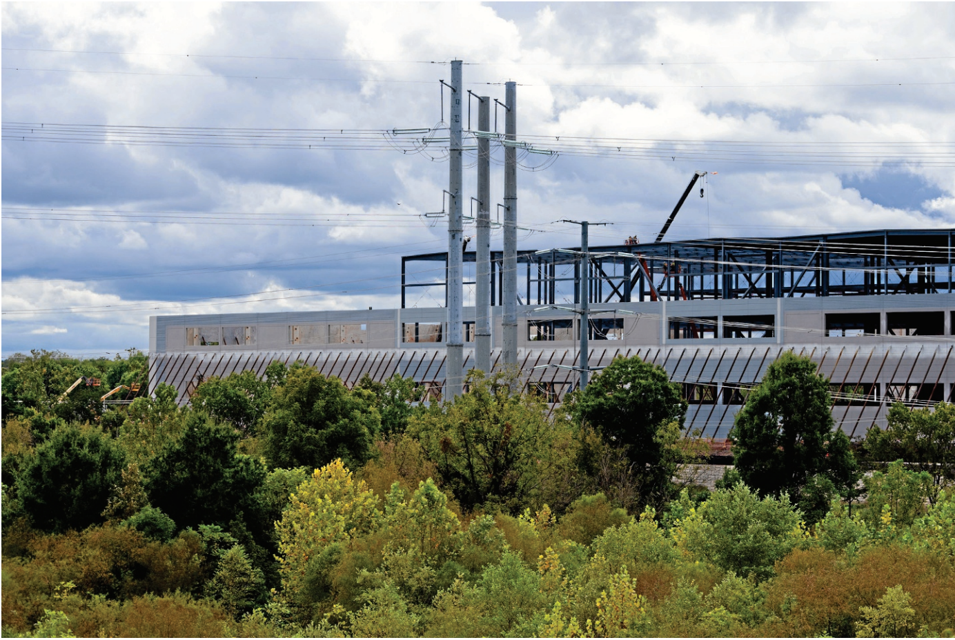
A data center is under construction in September in Virginia's Loudoun County.
