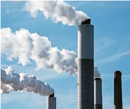
The EPA has eased limits on plants such as LG&E's coal-fired Mill Creek power plant in Kentucky. MATT STONE/USA TODAY NETWORK
