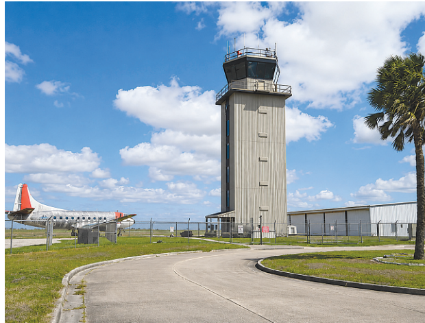
The Victoria Regional Airport air traffic control tower is undergoing a roughly $2.2 million rehabilitation project, with a $510,069 Federal Aviation Administration grant approved Monday covering 95% of the latest phase. (Lindsey Plotkin/Victoria Advocate)
