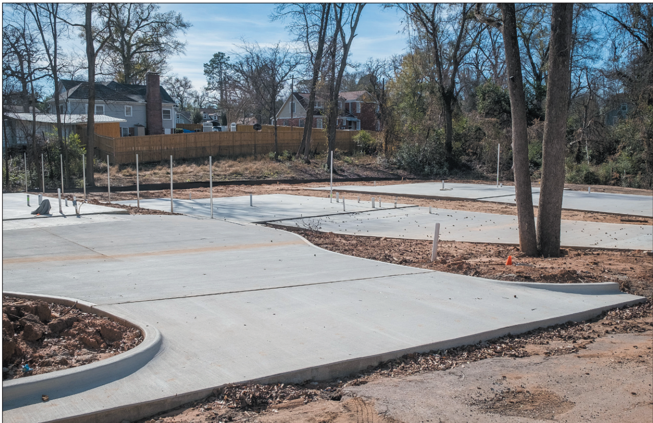
Foundation is poured for three future Habitat for Humanity of Smith County homes on W. Shaw Street in Tyler in 2022. (Les Hassell/Tyler Morning Telegraph File)
