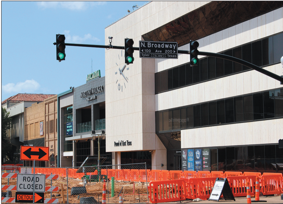
Infrastructure, sidewalk and roadway work will be ongoing on Broadway for the next phase of the project. (Jennifer Scott/Tyler Morning Telegraph)
