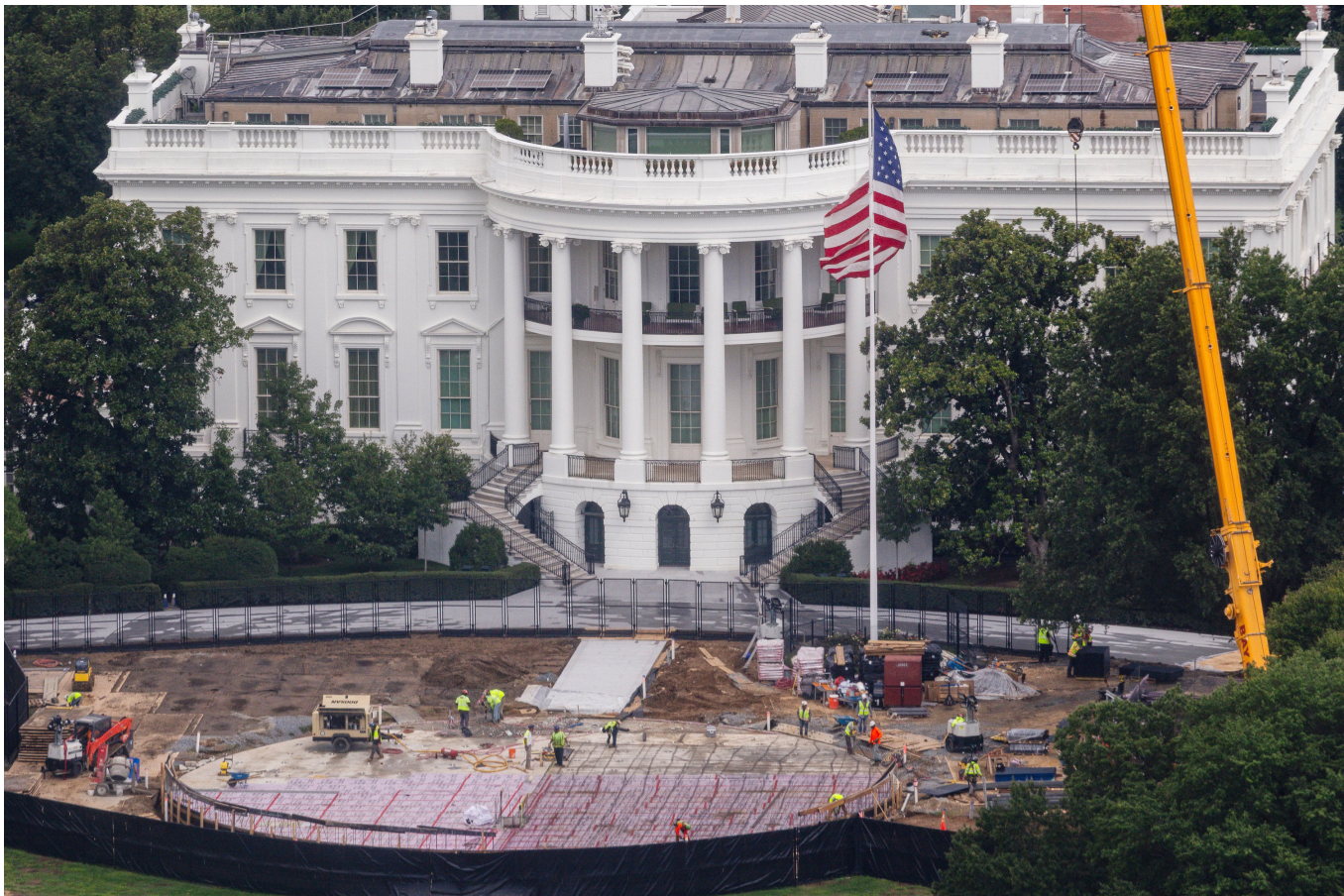
Construction continues on a helipad on the South Lawn of the White House on Wednesday in Washington. Workers used a jackhammer on the helipad, which no longer has the dark gray trim of a presidential seal. It’s unclear why the seal was removed. President Donald Trump’s administration says improvements are ongoing to meet White House needs. The president has said the helipad is necessary because new, more powerful Marine One helicopters damage the South Lawn grass. The helipad is part of a long list of renovations, including a new ballroom and changes to the Rose Garden and Oval Office. (AP Photo/Tierney L. Cross)
