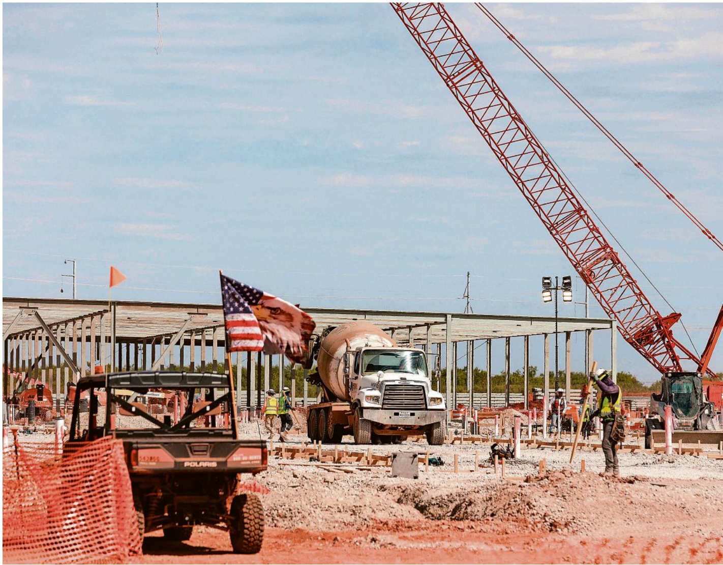
The steel frame of data centers under construction is visible during a tour of the OpenAI data center in Abilene in 2025. A total of eight data center buildings are planned to exist on the campus. SHELBY TAUBER/REUTERS
