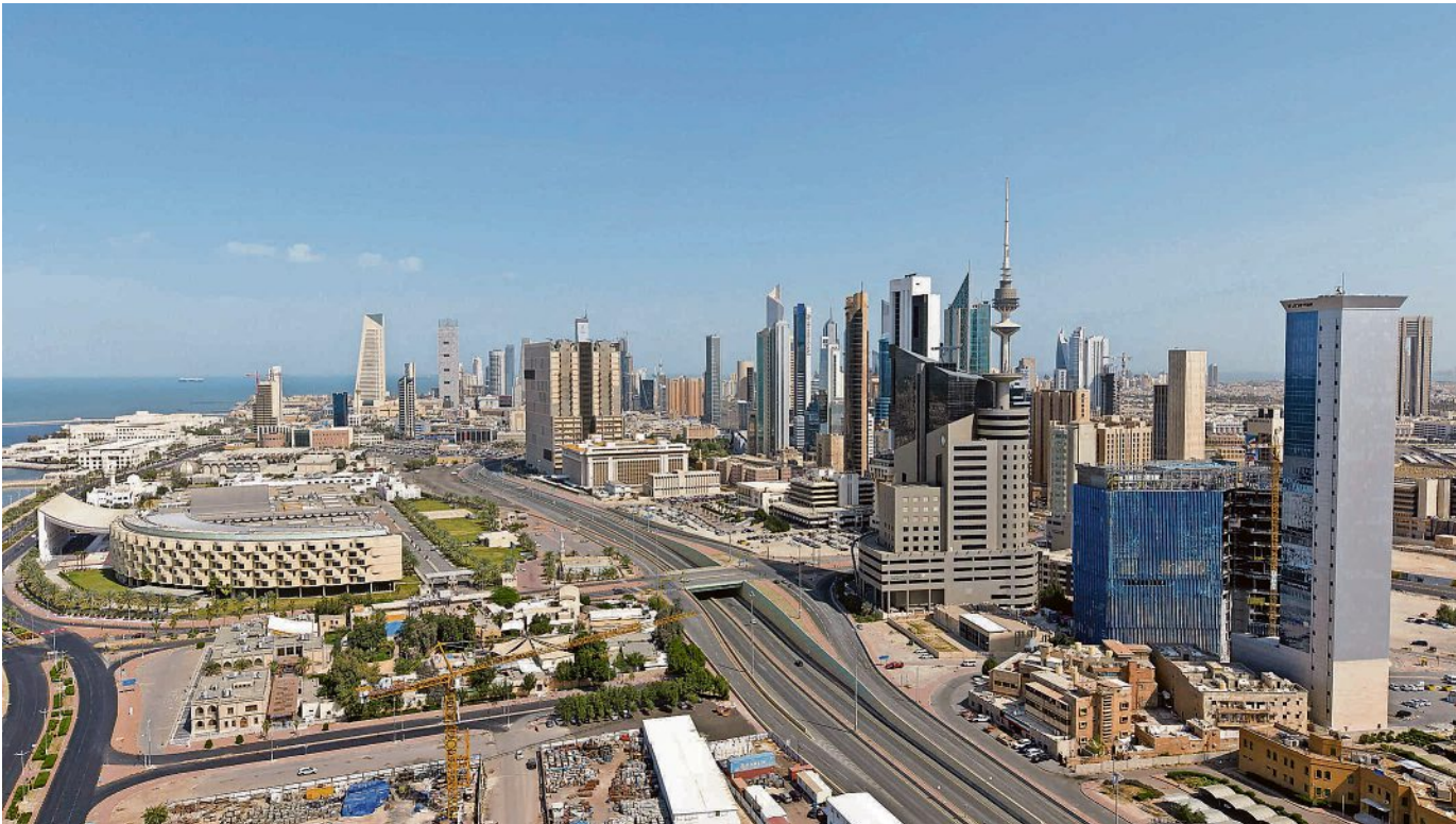
Authorities in Kuwait said one of its power generation and water desalination stations had been hit in an Iranian attack. STEPHANIE MCGEHEE/REUTERS FILE
