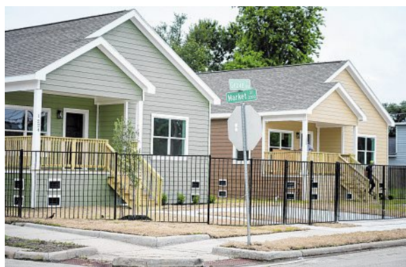
Jill Karnicki/Houston Chronicle Habitat for Humanity is having homes built inside a factory and shipped to Houston to cut costs.
