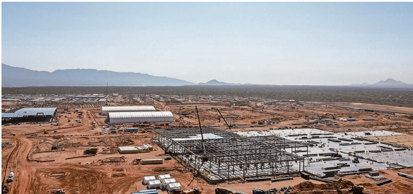
Buildings under construction at Oracle's Project Jupiter data center complex are seen in this drone image on Aug. 27 in Santa Teresa, N.M. PHOTOS BY OMAR ORNELAS/EL PASO TIMES
