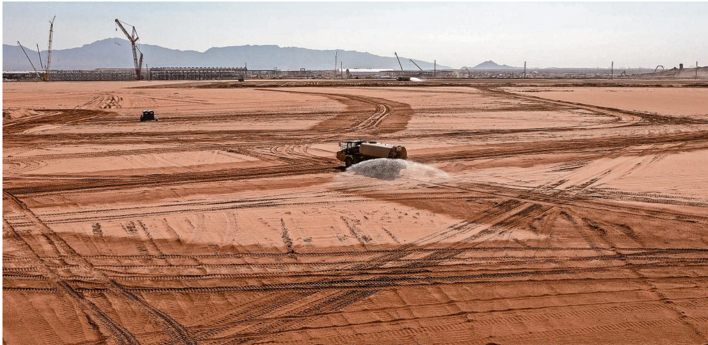
A water truck sprays water at the construction site of Oracle's Project Jupiter data center complex on Aug. 27 in Santa Teresa, N.M.
