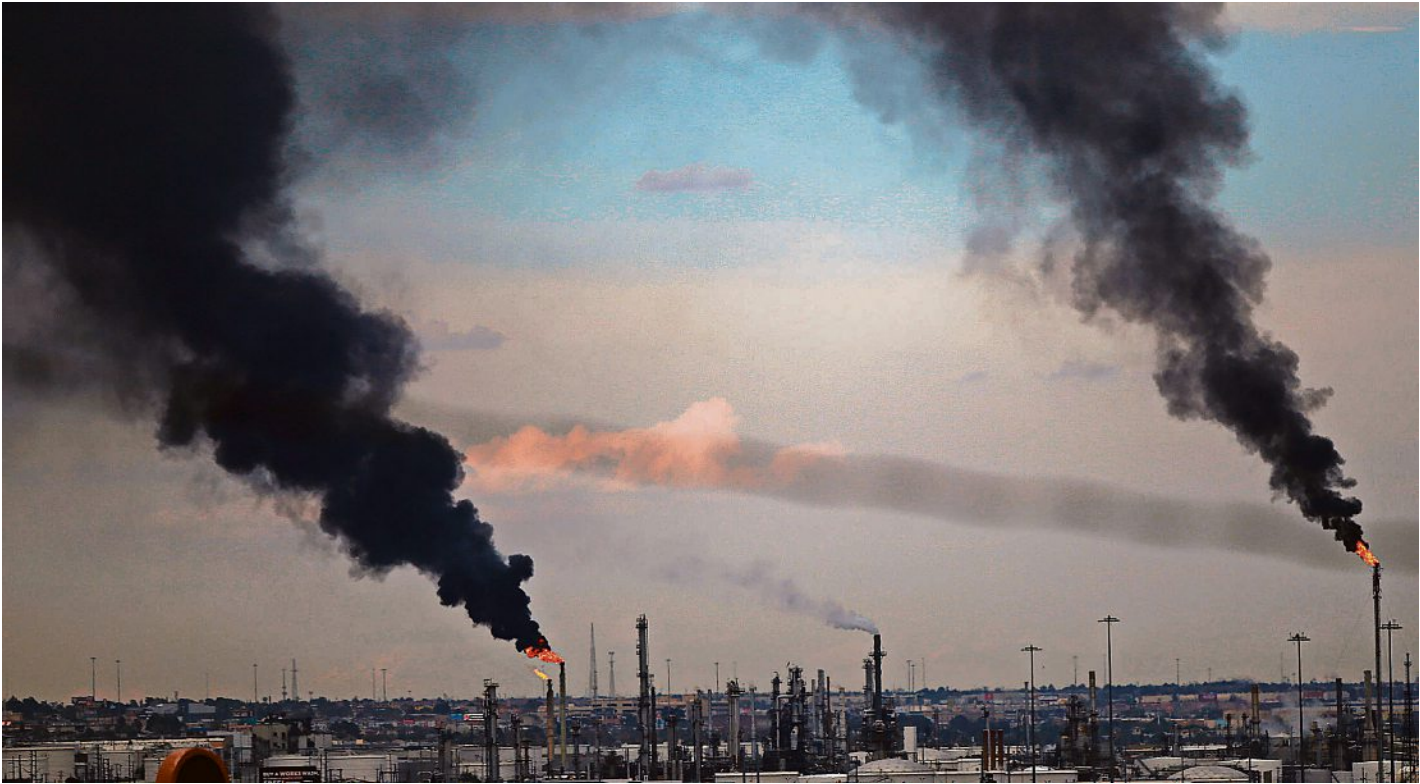
Black smoke flows from gas flares at the El Paso Marathon Petroleum refinery during a refinery problem on July 8, 2025. FERNANDO MENDEZ/SPECIAL TO THE EL PASO TIMES
