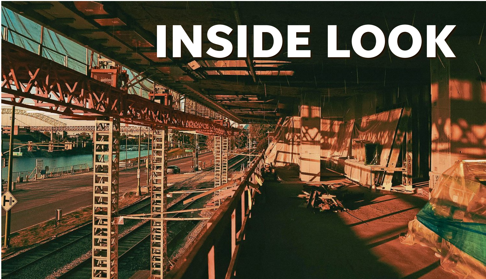
Work continues on the new Memphis Art Museum on Nov. 6 at Front Street and Union Avenue in Downtown. The museum is expected to open in December 2026. PHOTOS BY STU BOYD II/THE COMMERCIAL APPEAL
