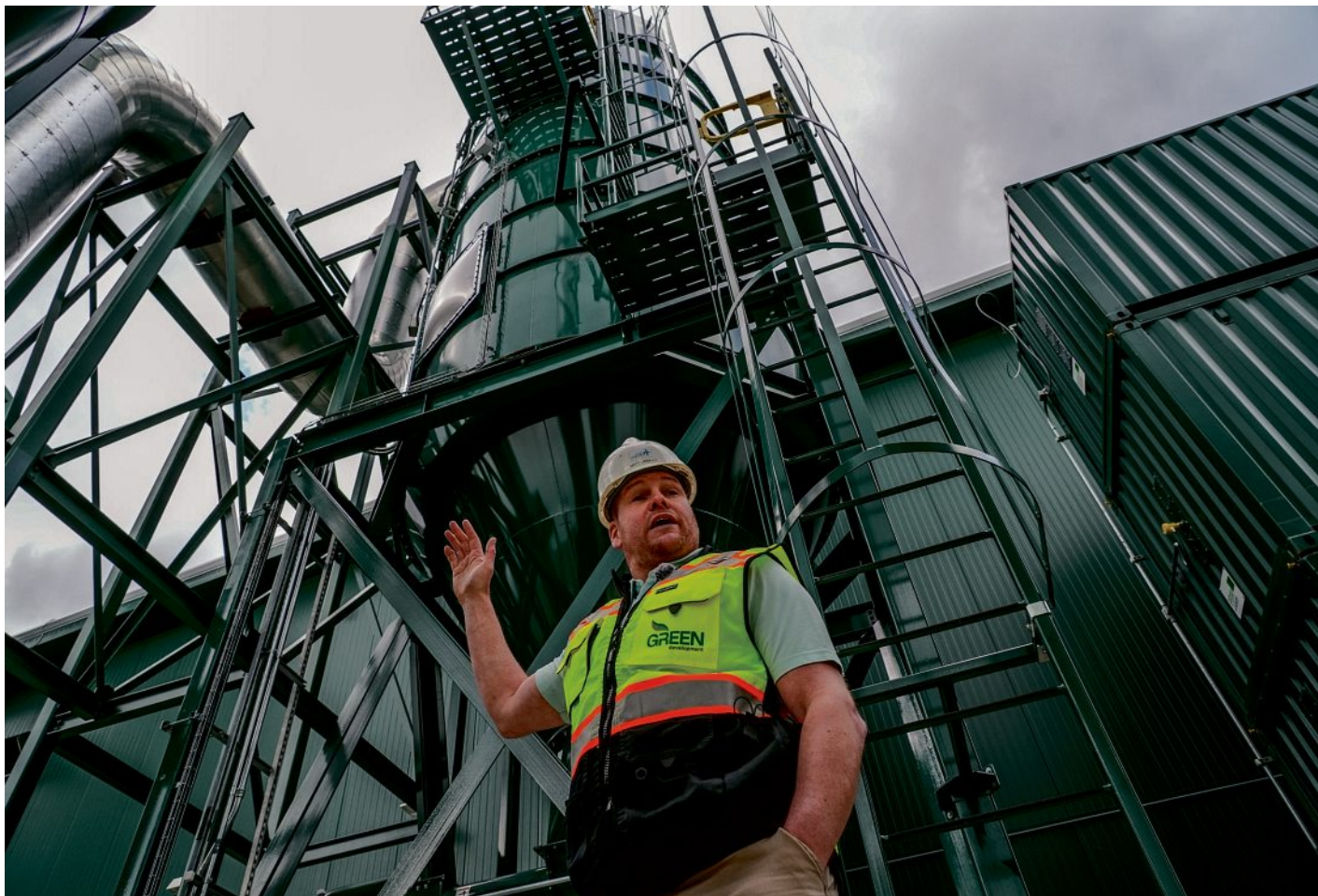
Matt Ursillo shows the Quonset Soil Solutions pyrolysis facility in North Kingstown on April 20. The plant uses a high-heat process to turn wood chips into a carbon-rich soil amendment. PHOTOS BY DAVID DELPOIO/THE PROVIDENCE JOURNAL
