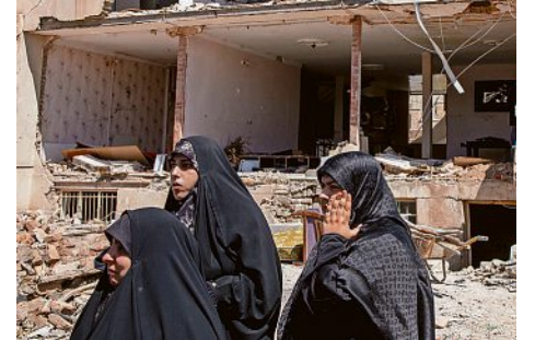
People stand outside a damaged residential building April 3 in Karaj, Iran. AJID SAEEDI/GETTY IMAGES
