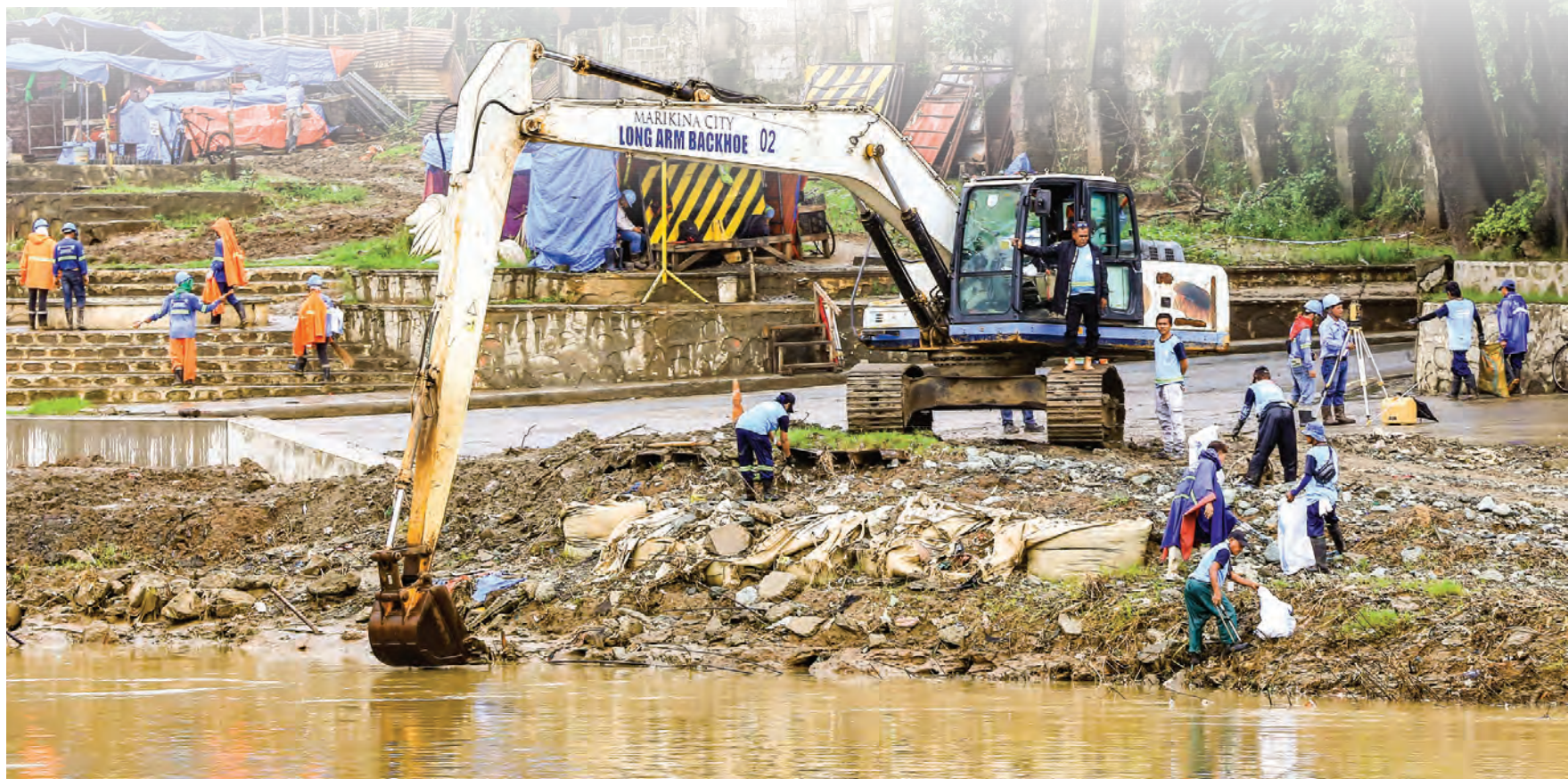
EFFICIENT SOLID WASTE, FLOOD MANAGEMENT — President Ferdinand R. Marcos Jr. (top photo, right) is joined by Department of Public Works and Highways (DPWH) Secretary Vince Dizon in inspecting the flood mitigation efforts being undertaken at the Marikina River (lower photo) by the ‘Estero Rangers’ on a rainy Monday, Sept. 7, 2026. Story on page 3. (Santi San Juan)
