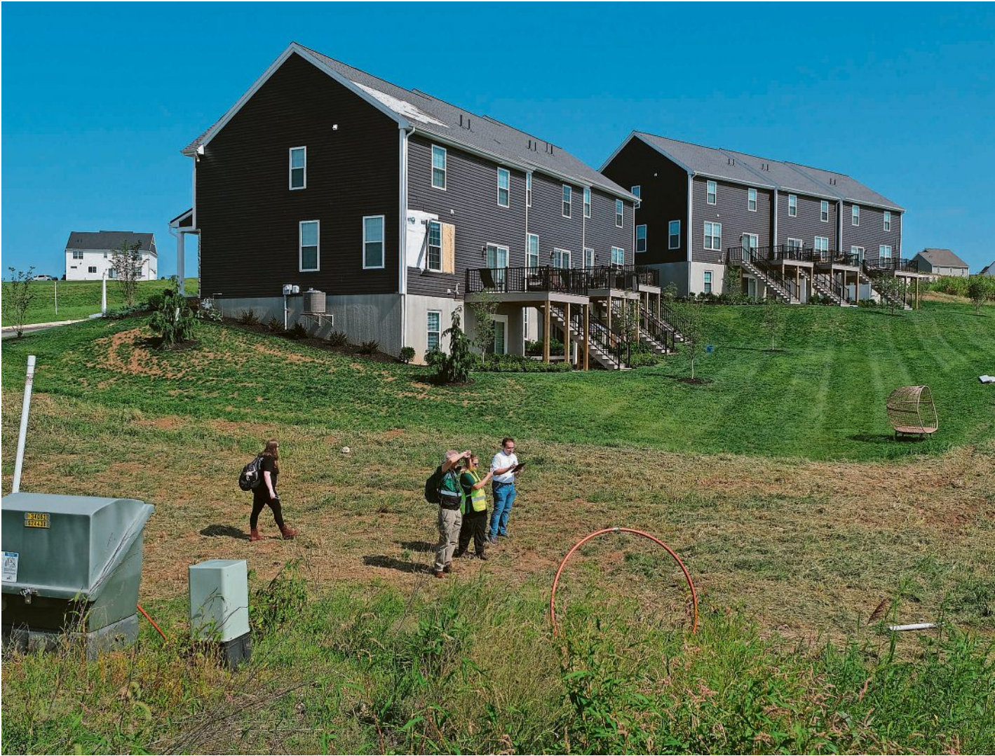
Officials begin to survey the damage from the storm that hit Eastern York High School and the surrounding areas on Aug. 20. MEREDITH WILLSE/YORK DAILY RECORD
