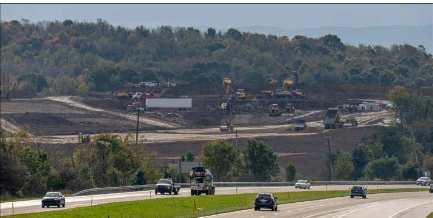
Work continues on asphalt plant site along Route 119 in East Huntingdon. (Louis B. Ruediger | TribLive)
