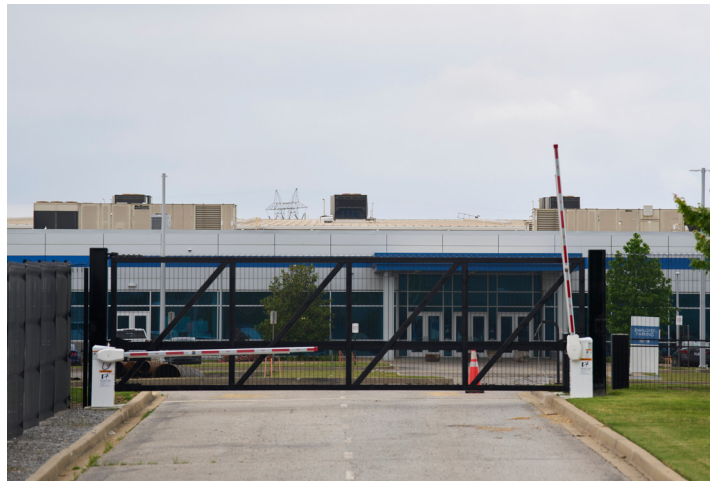
The xAI data center is seen, May 7, 2025, in Memphis, Tenn.
