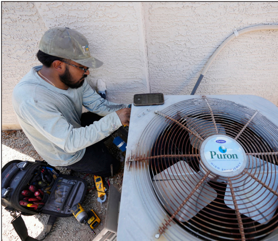
Total Refrigeration service tech Michael Villa works on replacing a fan motor on an air conditioning unit on July 19, 2023, in Phoenix. ASSOCIATED PRESS FILE
