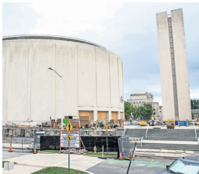
The State Museum, left, and the PHMC Tower that formerly housed the State Archives are part of the renovation.
