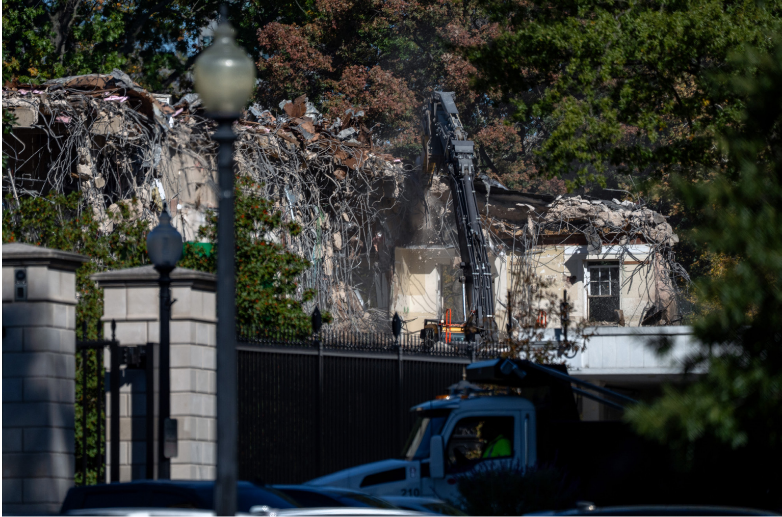
Demolition crews continue to dismantle parts of the East Wing of the White House on Wednesday. The work is part of the construction of a new ballroom, ordered by President Donald Trump. Peter W. Stevenson / Washington Post
