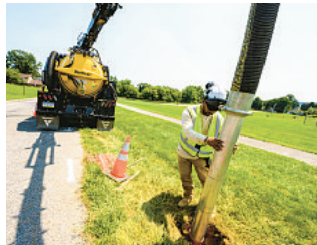
Jose Merino, a contractor for Comcast, uses a hydro-vac Tuesday in Bethlehem Township. Comcast is installing cable lines for internet and other digital service as it continues to expand into the Lehigh Valley.
