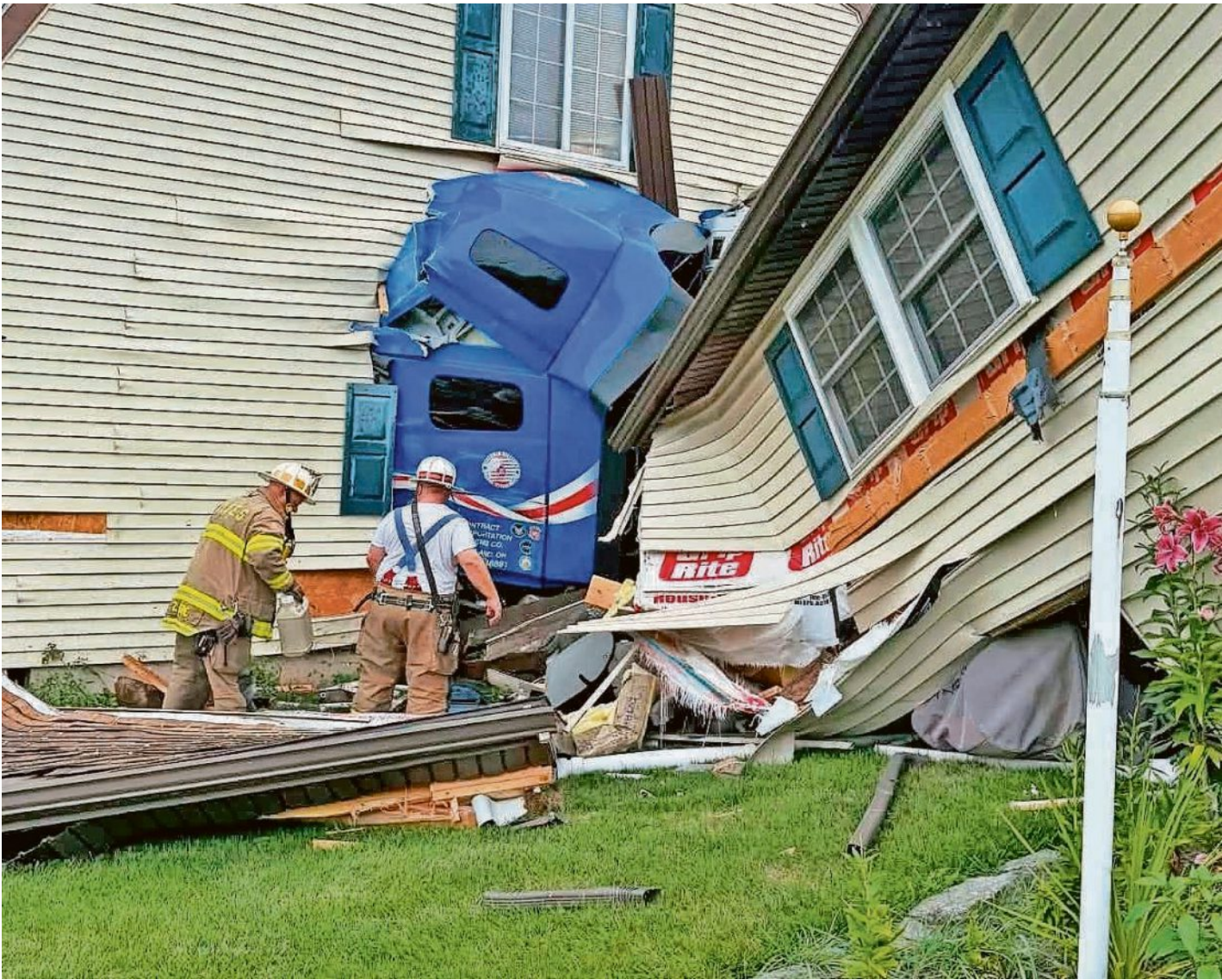
A tractor-trailer crashed into a garage in Swatara Township on Aug. 5, prompting an extended road closure on Route 72, according to a PennDOT spokesperson. IMAGE PROVIDED BY BUNKER HILL FIRE COMPANY
