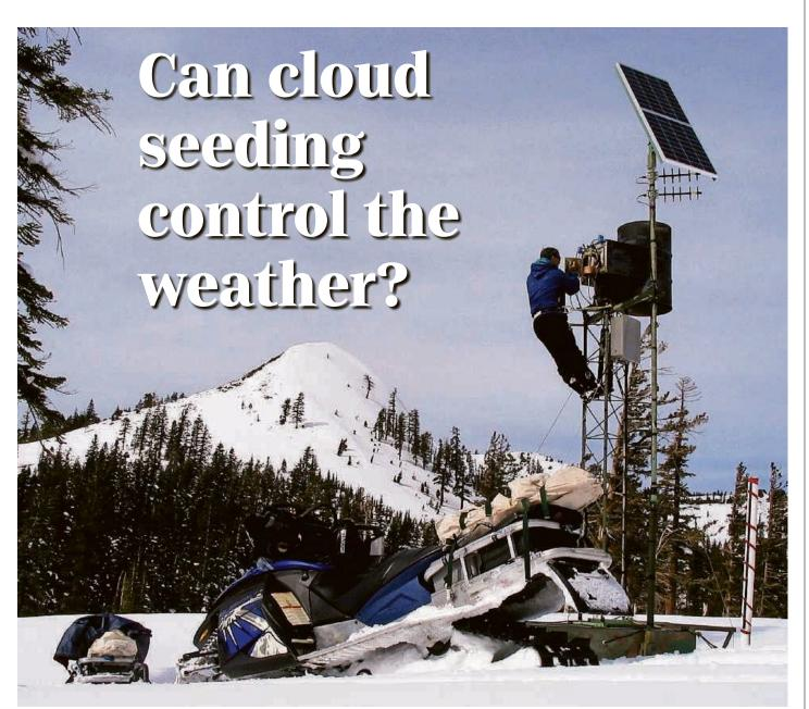
A technician works at a cloud-seeding generator high atop the Sierra. Five cloud-seeding generators seed storms with silver iodide particles, enhancing ice particle formation in storm clouds and boosting the snowpack for the Tahoe-Truckee area. JASON BEAN/RENO GAZETTE JOURNAL FILE
