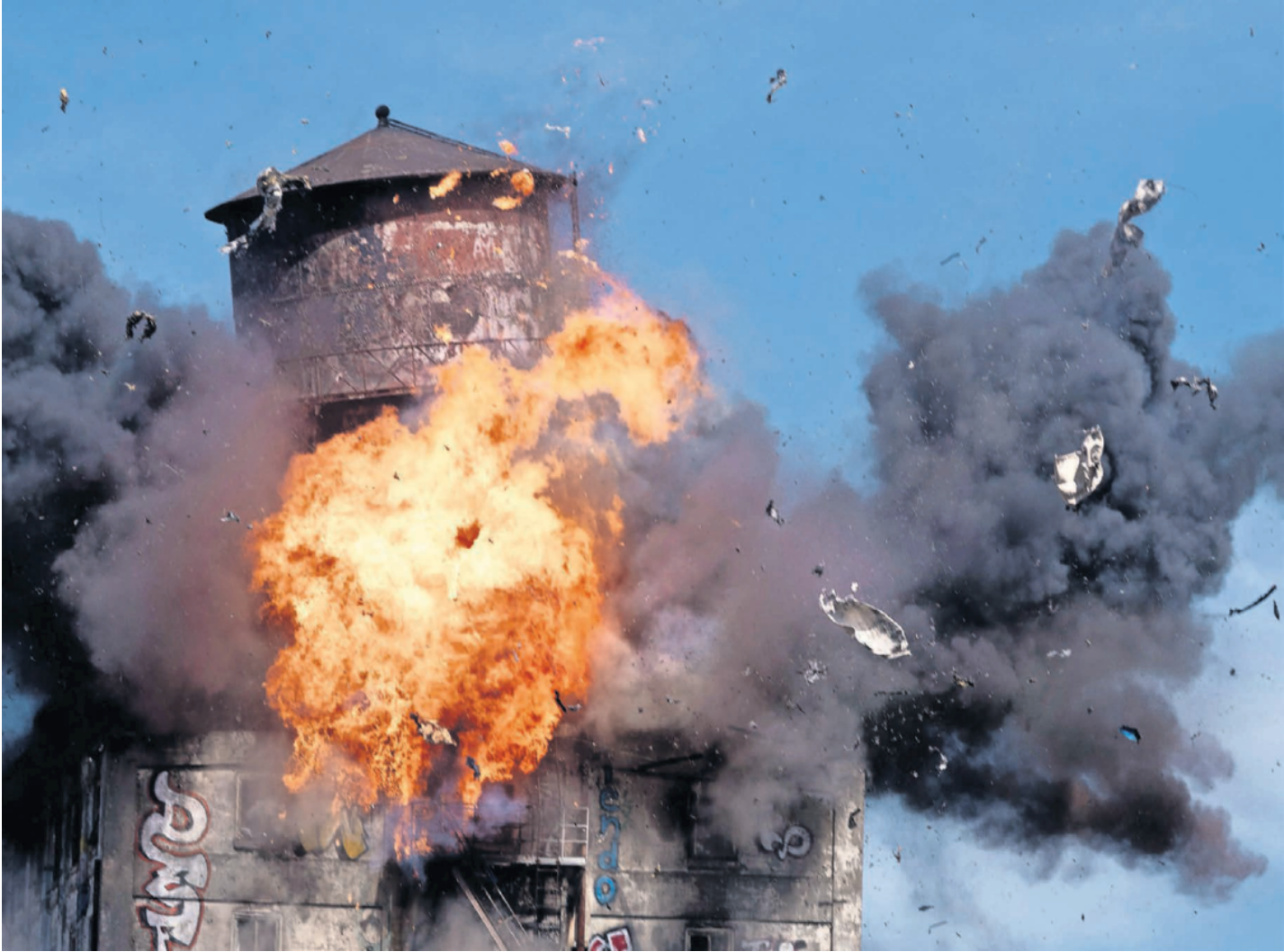
Demolition crews used explosives to bring down the water tank at the top of the Centennial Mills wreckage, the first step toward demolishing the structure after a fire. Photos by Beth Nakamura, staff
