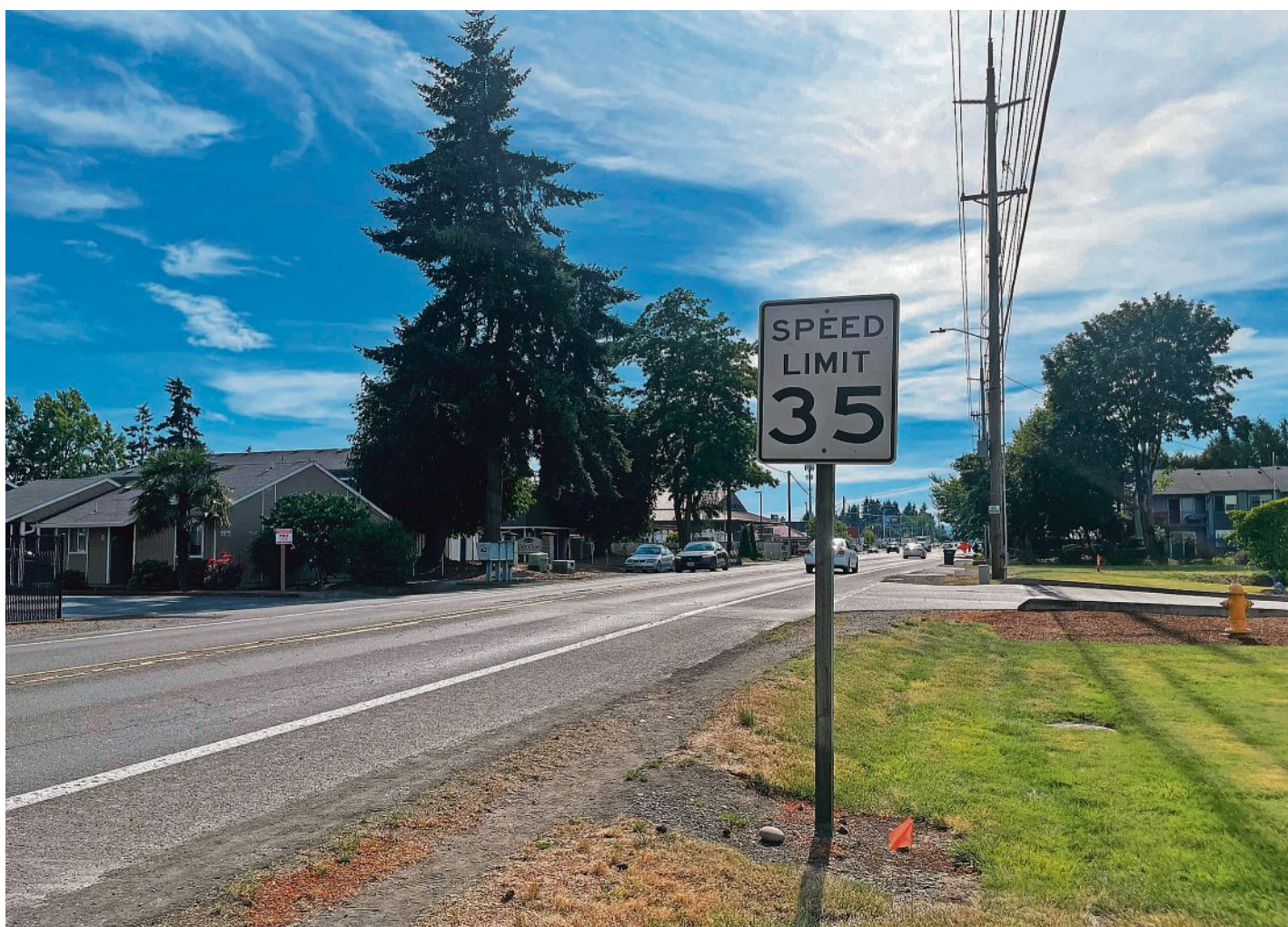
State Street will be widened to three lanes and a sidewalk will be added on the south side from The Yard Food Park to 46th Avenue. BILL POEHLER/STATESMAN JOURNAL
