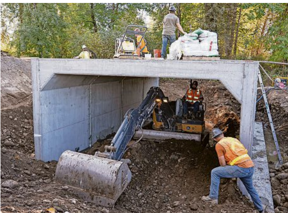
Construction workers build culverts to help with habitat restoration at the Confederated Tribes of Grand Ronde's Chahalpam property. KEVIN NERI/STATESMAN JOURNAL
