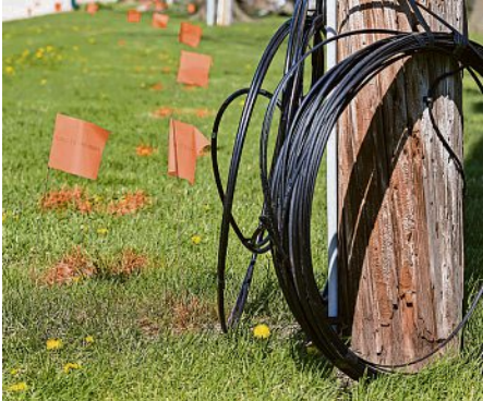
Orange flags signal the upcoming installation of an underground communication line. Different color flags have different universal meanings in excavating and utility world. Learn them and you'll know what kind of project is happening in your neighborhood.
