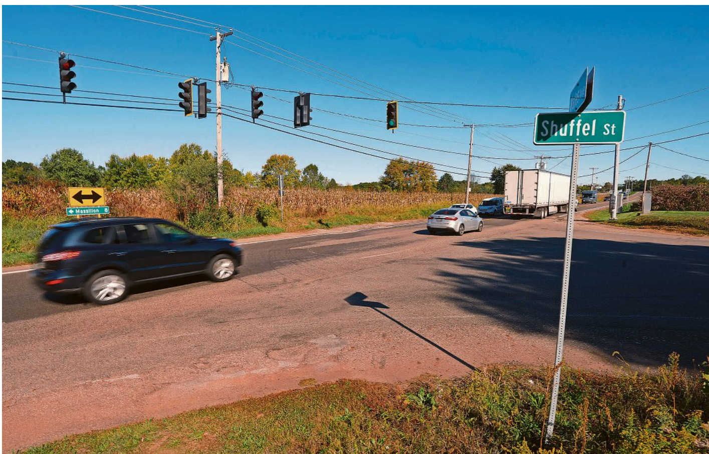
The Ohio Department of Transportation plans to add a roundabout at the intersection of Wales Avenue NW and Shuffel Street NW in Jackson Township. PHOTOS BY KEVIN WHITLOCK/MASSILLON INDEPENDENT
