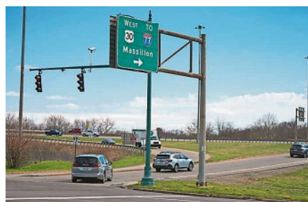
The Ohio Department of Transportation will spend $12.8 million this year to resurface U.S. Route 30 and state Route 172 in Canton and surrounding areas.
