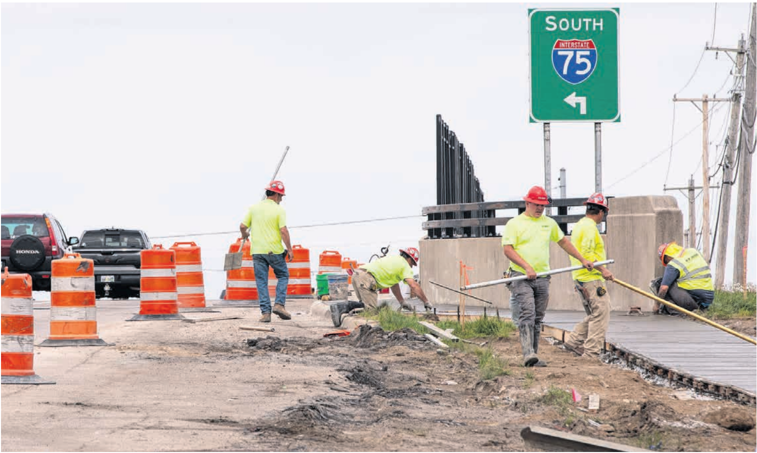
Construction workers smooth out sections of concrete April 16 during a sidewalk installation on the West Main Street bridge in Troy that crosses Interstate 75. One area of juxtaposition between the two candidates for Ohio governor is within the building and construction trades councils. BRYANT BILLING / STAFF
