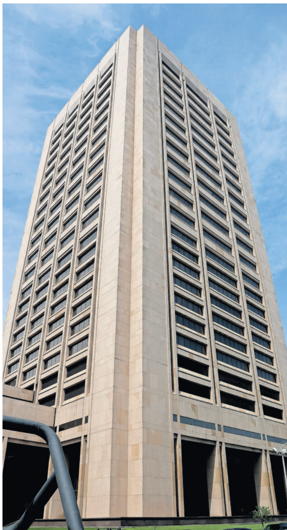
The Courts Tower at the Justice Center downtown is a 26-story building that houses criminal courtrooms, the prosecutor's office, clerk of courts and municipal courts. The Plain Dealer
