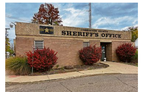
The former Coshocton Justice Center building in the 300 block of Chestnut Street will be demolished with leftover funding from a state grant in 2025. The plan is to create a parking lot for the Coshocton County Courthouse and free up parking along Main Street.
