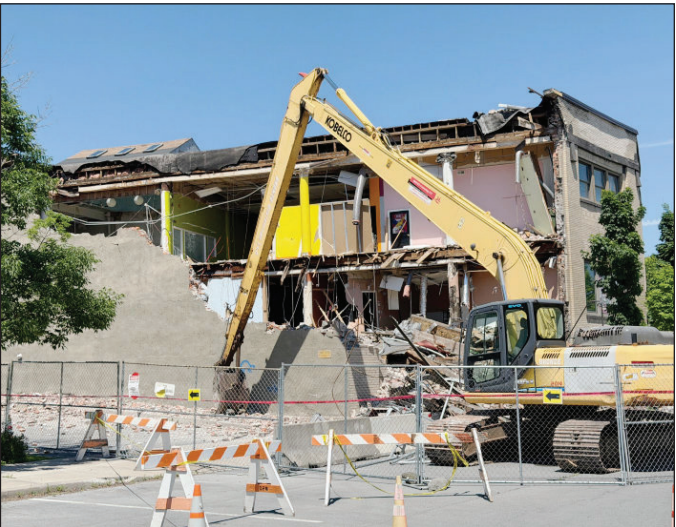
Demolition progressed on J.B. Wise Place in Watertown in June. Alec Johnson/ Watertown Daily Times
