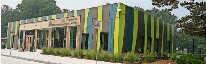
The Maplewood Nature Center in Maplewood Park in Rochester has been open for R-Camp since July 6 and opens to the public July 21. Work outside the facility, including revitalization of the nearby pond area, remains ongoing.
