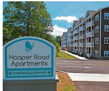
The CDS housing community features 80 apartments, a fitness room, computer lab, community room, and two laundry rooms.
