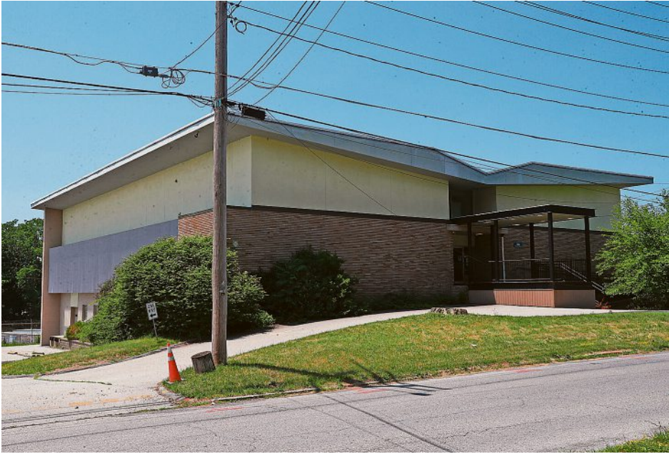
The property at 26 Oakley Street in the City of Poughkeepsie on June 29. Dutchess County and the City of Poughkeepsie are working towards an agreement for the property to become a homeless shelter.
