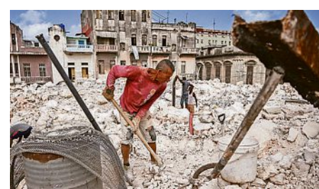
A man collects materials to sell from the rubble of the National School of Design in Havana on March 16. Cuba has struggled with blackouts and energy shortages.
