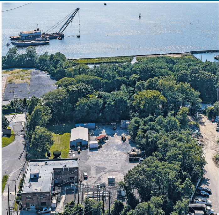
The property for a proposed substation for the Propel NY Energy cable project in Glenwood Landing, looking toward Hempstead Harbor.
