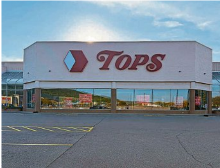
A look at the former Tops Market store in Big Flats, which will not reopen after sustaining fire damage in August. JEFF SMITH/CORNING LEADER
