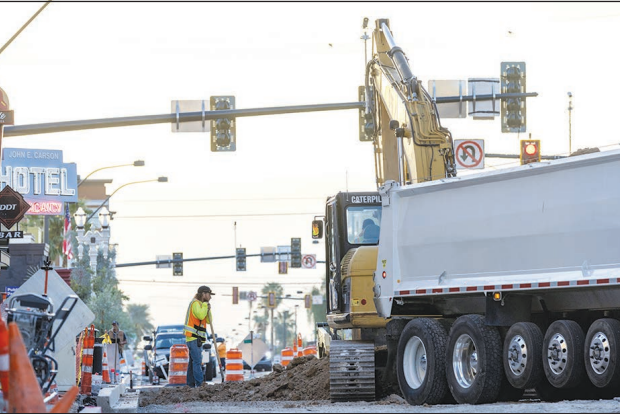
The construction work taking place on Carson Avenue is part of the $378 million Maryland Parkway improvement project.
