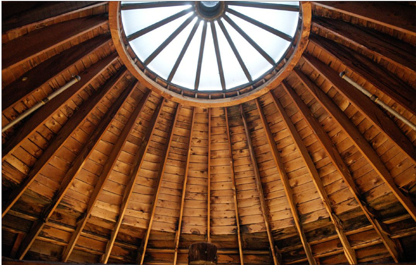
Staining of the wooden structure shows from water leaking under the copper cladding of the Kimball Public Library cuppola in Randolph on Thursday.
