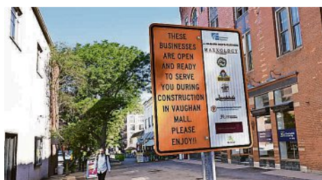
Construction at Vaughan Mall, seen June 16, is creating a wider space for pedestrians in Portsmouth. DEB CRAM/SEACOASTONLINE
