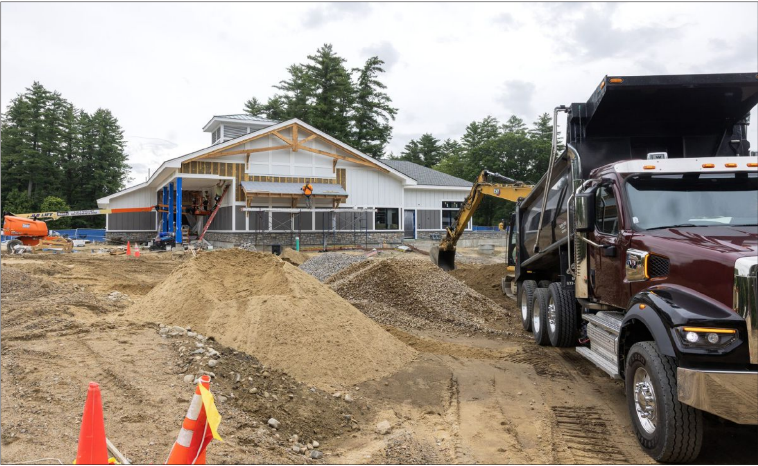
Construction and site workers at Beaver Meadow Golf Course work around each other as progress is being made on the project on Wednesday.
